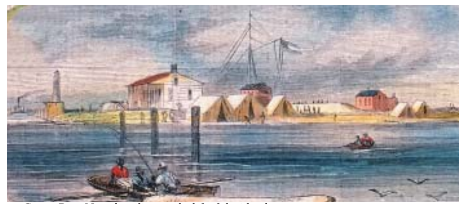
Grants Pass. Note the pilings to the left of the island.
